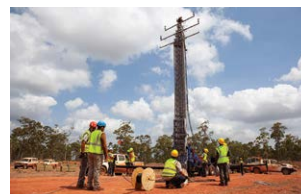
Wind tower installation
