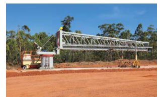
Medium Mobile Launcher assembly completed.
